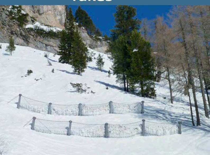
Flexible-net snow rakes are similar to snow nets as they are installed in potential initiation zones to prevent avalanches from developing.
