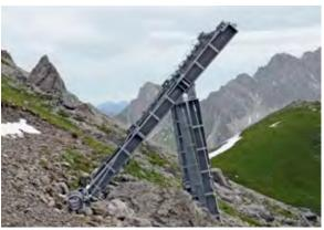
Compared to avalanche dams, catchment fences require less construction space. Thus, a larger area is available for the controlled interception and deposition of the avalanche.
