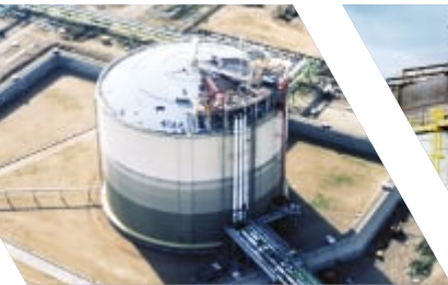
Containment dikes for ammonia tanks - Montoir (France)
