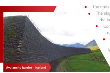
• The embankment slope can be steepened up to 90°;
